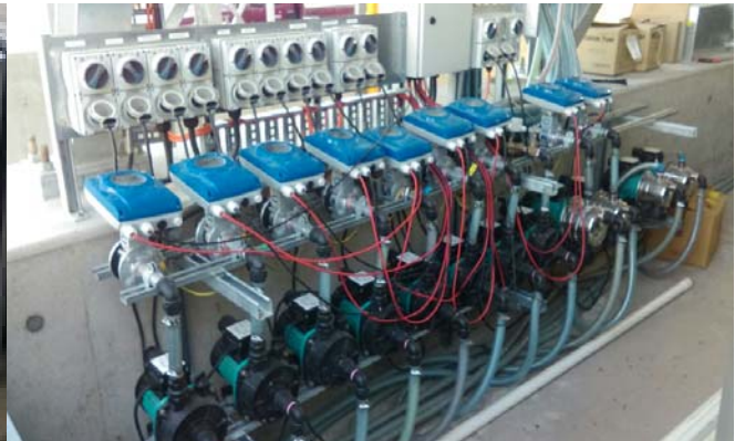
KMS502-25F 25mm flowmeters install
