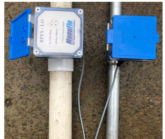
RPFS-LOD installed on a 50mm PVC pressure pipe line and 25mm galvanised steel pipe, using PVC50 and GAL25 adaptors.
